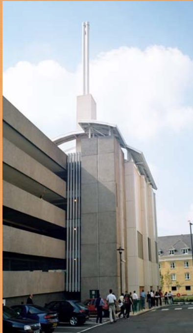
Figure 2: Woking Borough Council Town Centre Combined Heat and Power Plant
